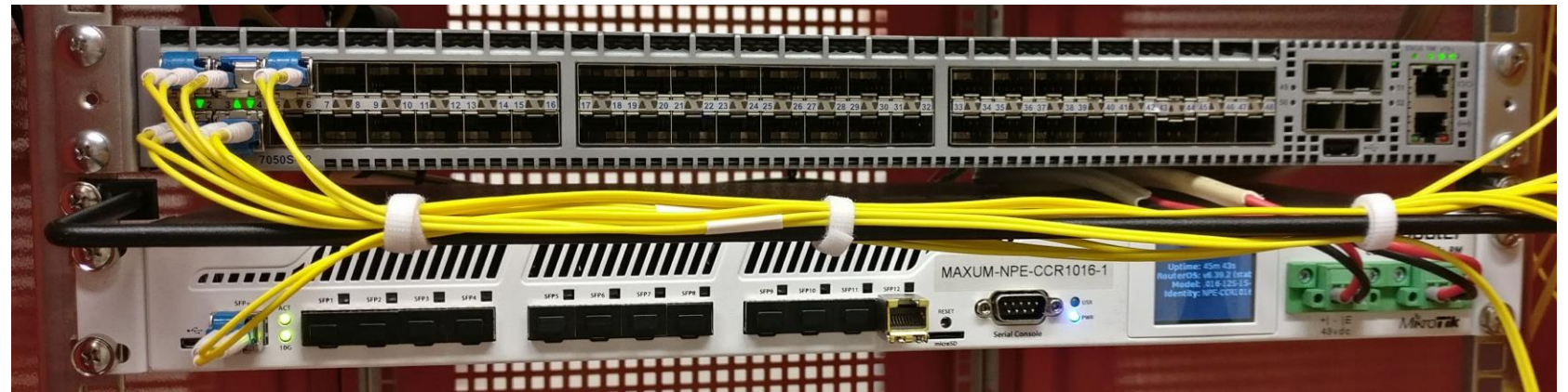
Mikrotik CCR1016 with Dual 48VDC Conversion in Napier Exchange
